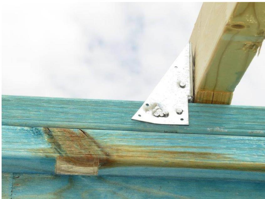
Photo 1: - Example of framing anchor not correctly nailed off and fixed to ribbon plate only
